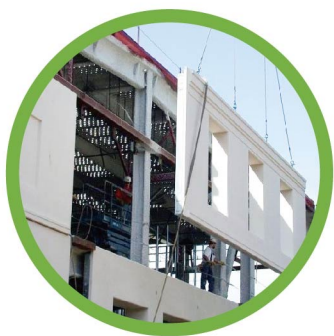
Precast concrete sealing
